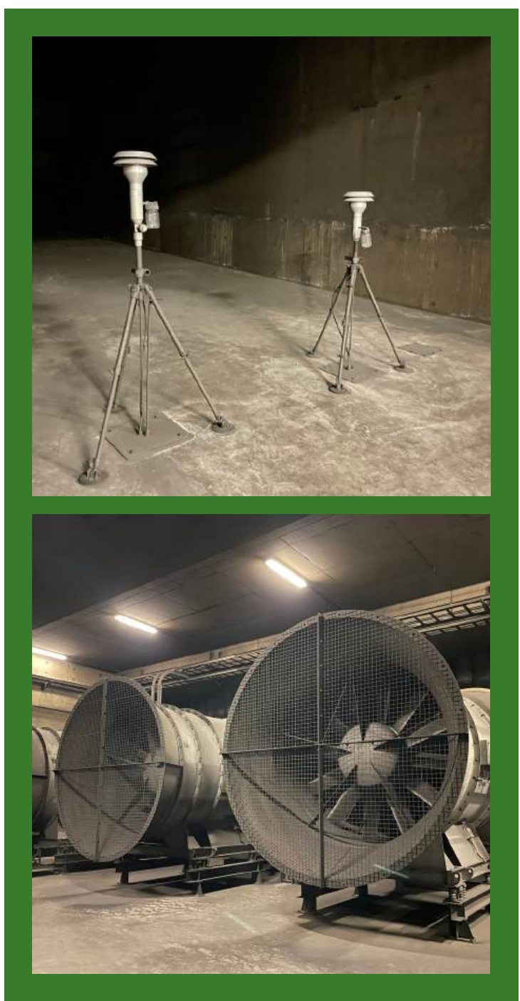
Pictured below: particulate matter sensors inside the stack (top); exhaust fans to extract tunnel air through the stack (bottom)
