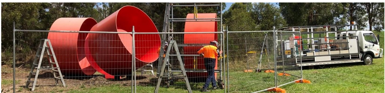
Image 12: Red Rings during renovation
