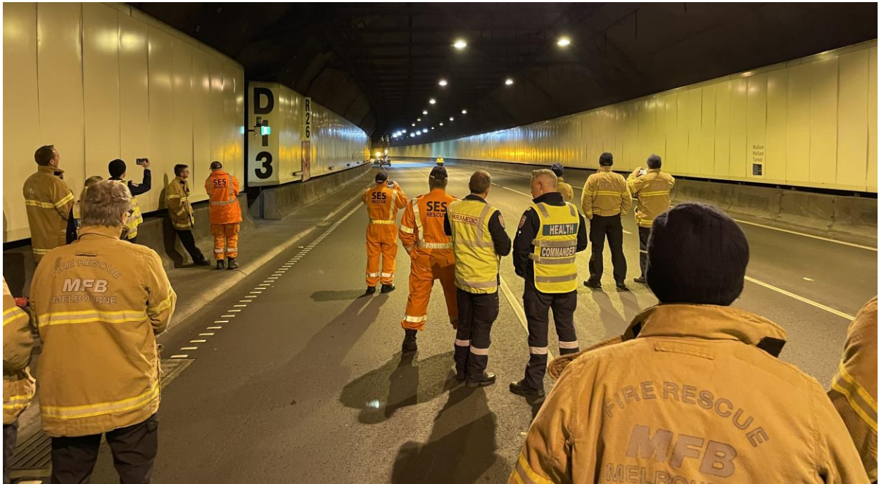
Image 19: Emergency services personnel about to watch a demonstration of the fire suppression deluge system (22 May 2021)
