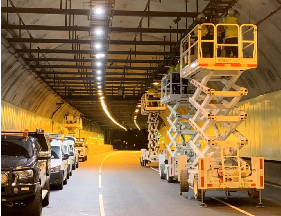
Image 4: New LED lights (white) being installed in an EastLink tunnel
