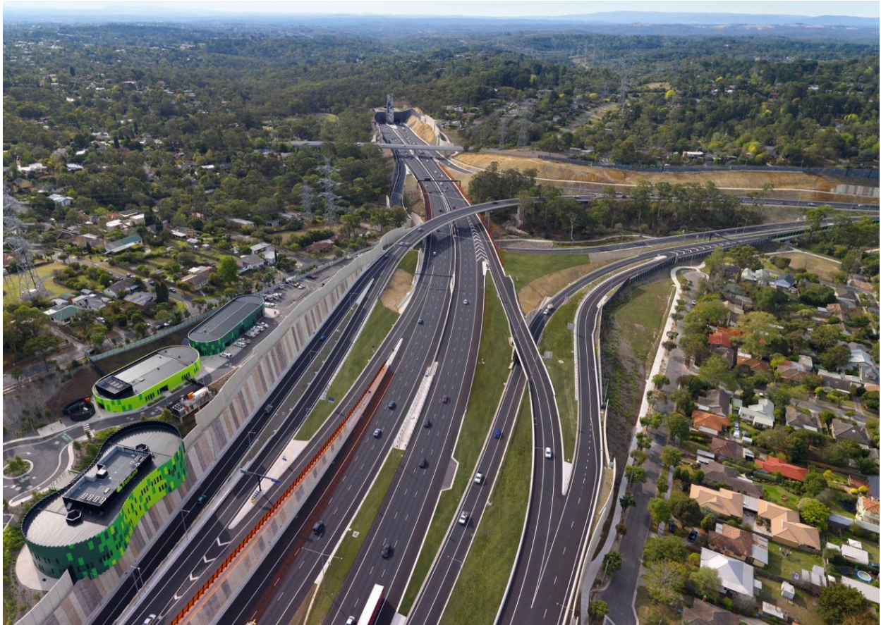
Image 1: The EastLink operations centre in Ringwood, adjacent to EastLink with the EastLink tunnels in the background
