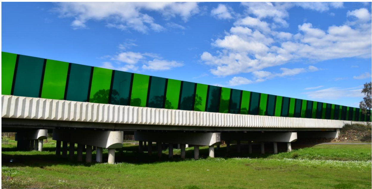
Image 43: EastLink removes graffiti promptly to maintain asset aesthetics (bridges, noise panels)
