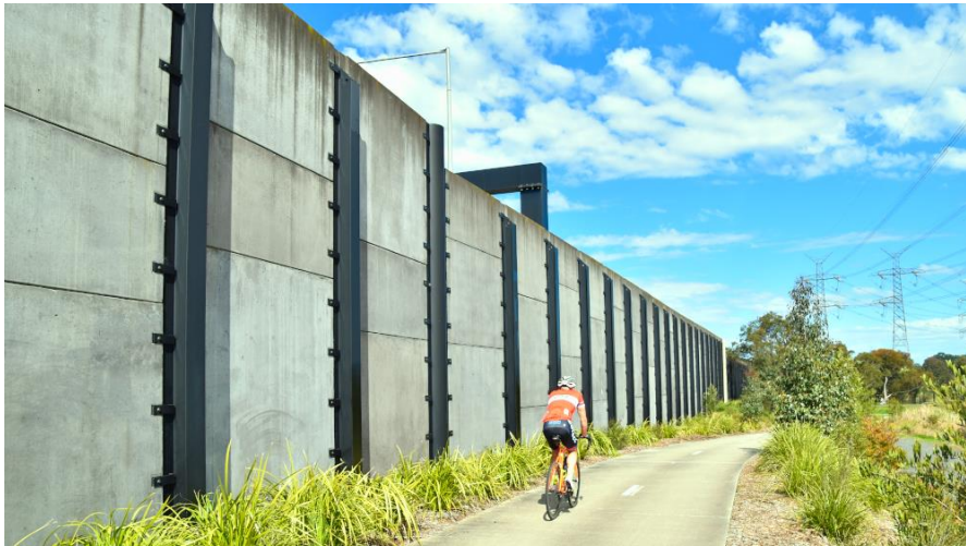
Image 42: EastLink removes graffiti promptly to maintain asset aesthetics (noise panels)
