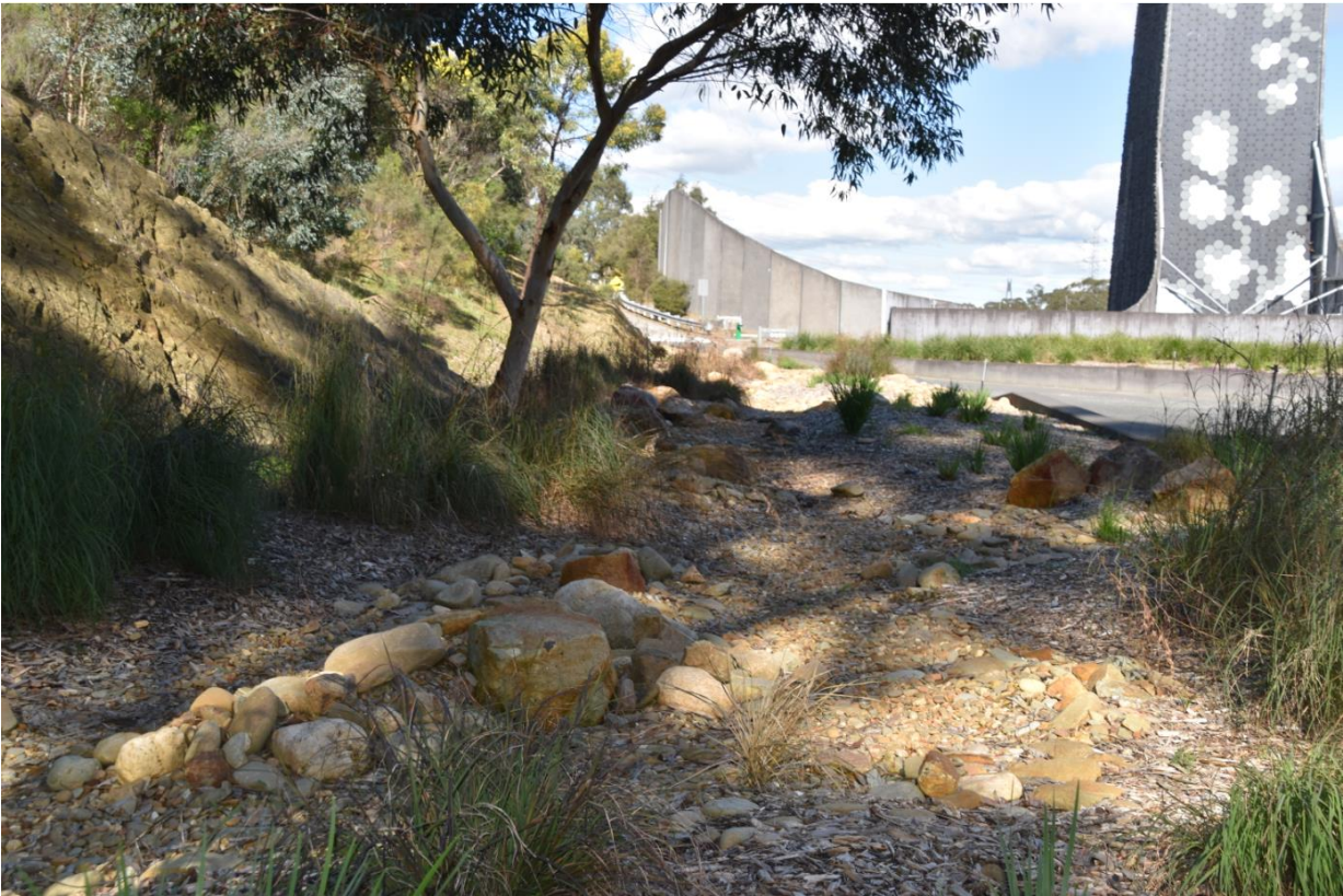
Image 41: Recent view of the garden area showing the new naturalistic creek bed drainage swale
